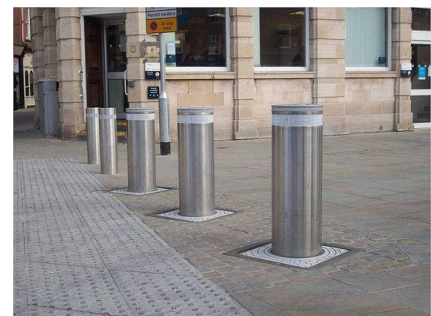
Figure 44 Retractable bollards and textured concrete help define temporary pedestrian zones
